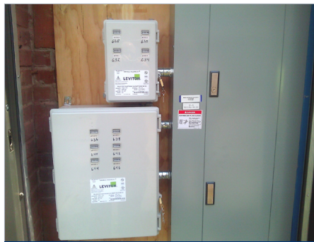
After: Odometer-like display on VerifEye submeters can be read at a glance.
