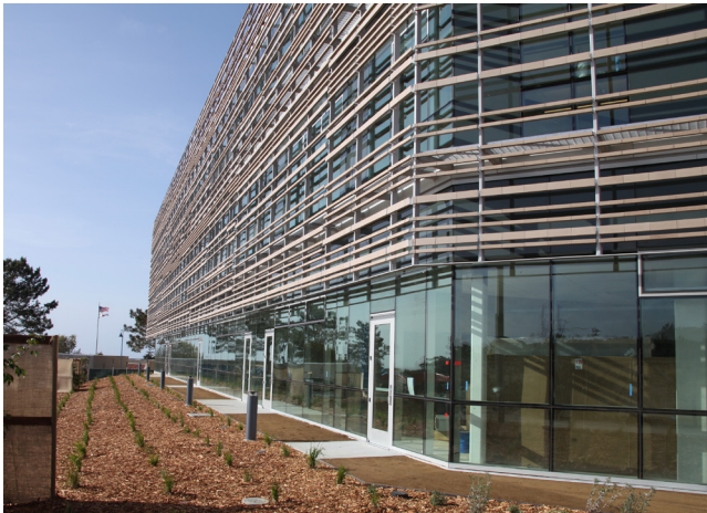
New CSU Monterey Bay Business and Information Technology Building.
