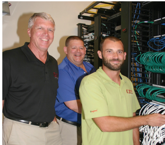
Double checking the installation.
