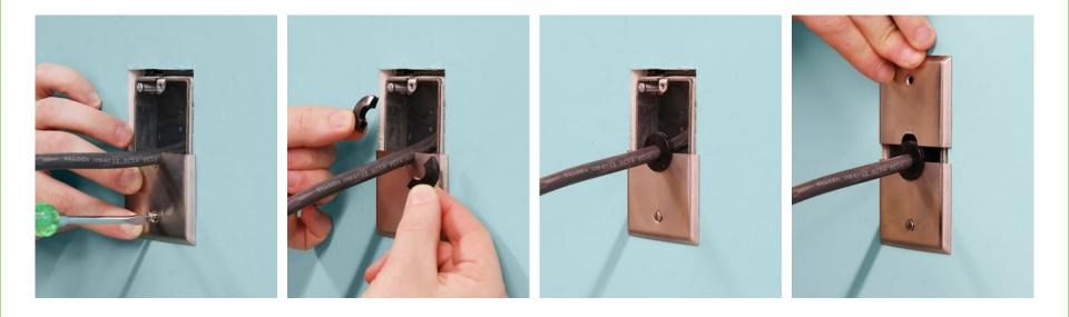
With the cord coming out of the box, screw the bottom half of the wallplate into the wall box Place both halves of the gasket around the cord and fit the assembly into the center hole of the wallplate
