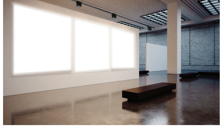
Stealth LED luminaires cast wide, rectangular-shaped beams of light. They are specifically designed to provide superior uniformity for a clean, consistent, and shadow-free appearance.
