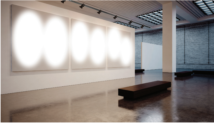
Cylindrical track fixtures cover a wall with pools of light. They contain hot spots and gaps with uneven distribution.
