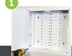
Loosen top two screws. Remove bottom two screws and existing metal door.
