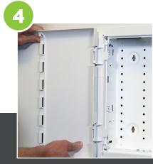
Snap Vented Hinged Door onto hinge.
