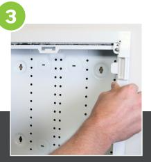
Hang Trim Ring or Vented Cover and screw in place (Cover installation is complete).
