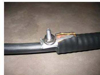
Ensure that the top and bottom plates compress onto the armor only and not the heat shrink or outer jacket.
