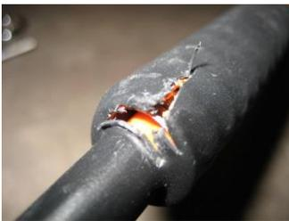
2. Using the Cable Sheath Knife, make a slit in the heat shrink (if present) and outer armor's jacket that is perpendicular to the cable. Expose the armor to an appropriate length to accommodate the bonding clamp being used.
