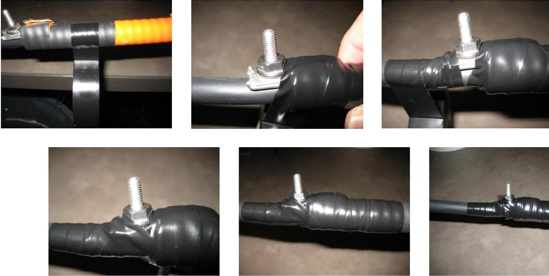
Ensure that the bonding stub and nut are not covered with tape as this will negate the bonding function.
