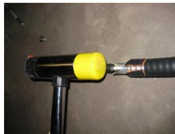
Use the mallet to gently insert the bottom plate under the armor. Make sure the jacket of the fiber optic cable is not damaged.
