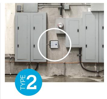
**Type 2 SPDs:** Intended for installation on the load side of the service equipment. Generally serve a branch circuit and protect against residual lightning energy, motor driven surges and other internally generated surges.
