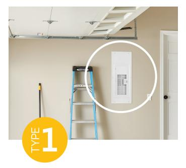
**Type 1 SPDs:** Intended for installation between the secondary side of the service transformer and the line side of the service equipment, as well as the load side. Protect against external surges caused by lightning or utility capacitor bank switching. Type 1 devices can automatically be used in Type 2 applications.
